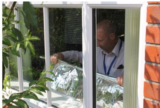
United Kingdom - Figure 15: Advisor installing a reflective radiator panel
