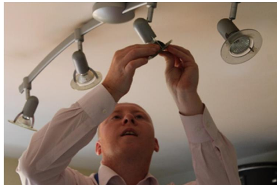
United Kingdom - Figure 16: Advisor installing an LED
